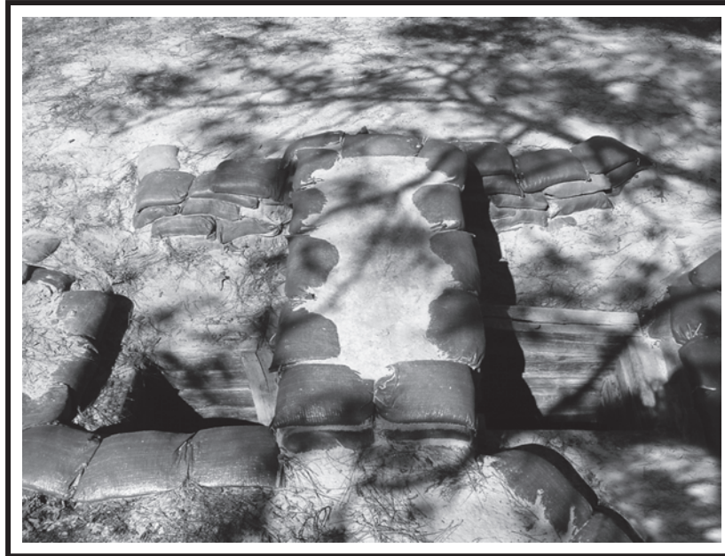
Figure 6-20. Machine gun fighting position with OHC.
