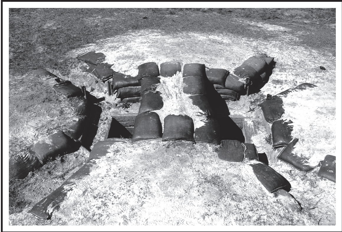
Figure 6-15. Two-man fighting position with built-up OHC (Stage 4).
